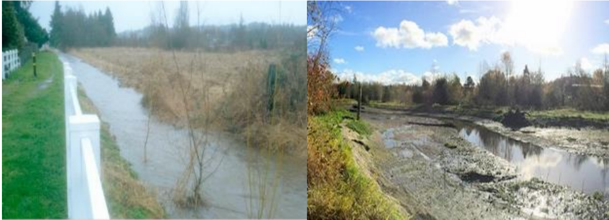
Figure 20. These photos show the creek before restoration (left) and after restoration (right). The left shows that the creek had become essentially a ditch. The restored portion on the right shows a wider channel with an associated freshwater wetland floodplain that creates salmon habitat, reduces flooding, and improves water quality. (Photo Source)
