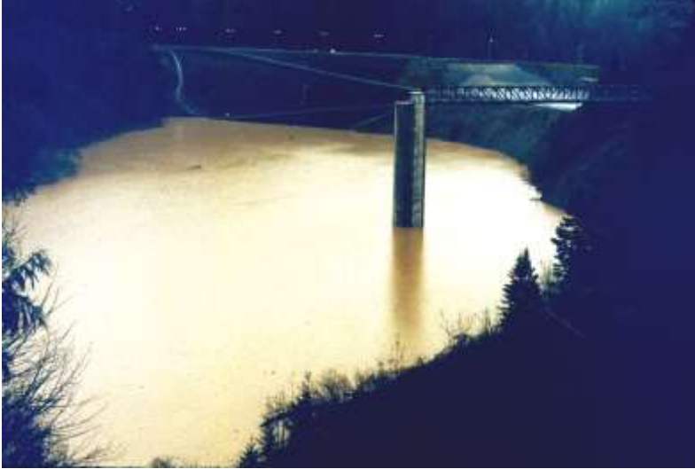
Figure 7.13 – Mud Mountain Dam during flood storage in February 1996
