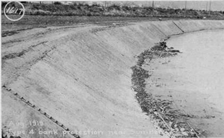
Finished Bank Slope at Sumner, Type No. 4
