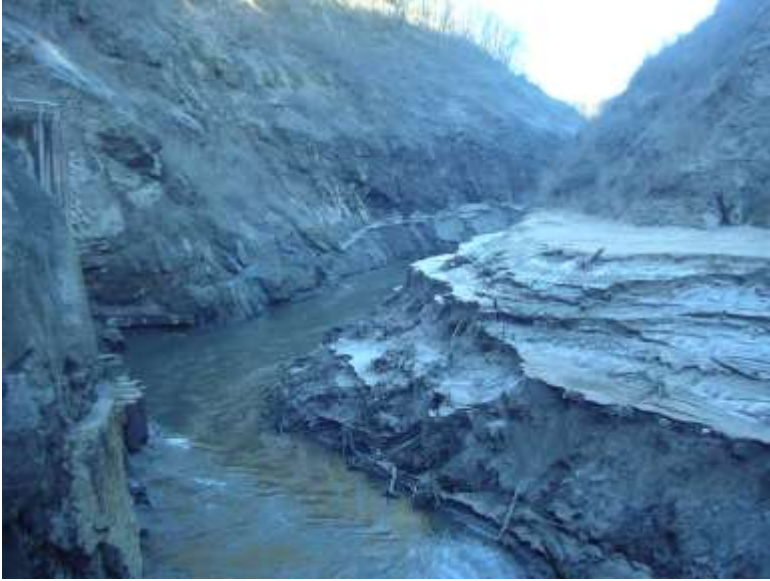
Figure 7.15 – White River flow through sediment deposited in MMD reservoir
