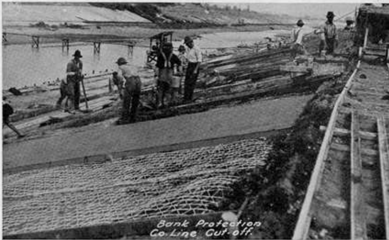
Paving Bank Slope with Concrete
