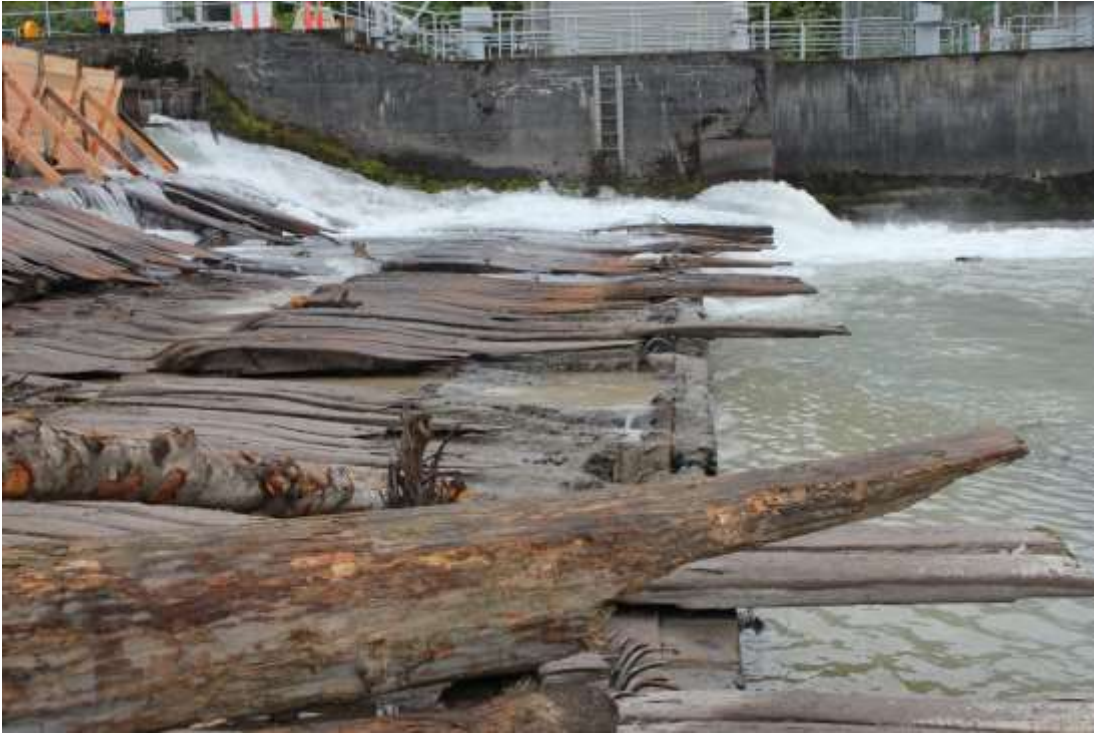
Figures 7.19 and 7.20 – Buckley Dam apron and foundation
