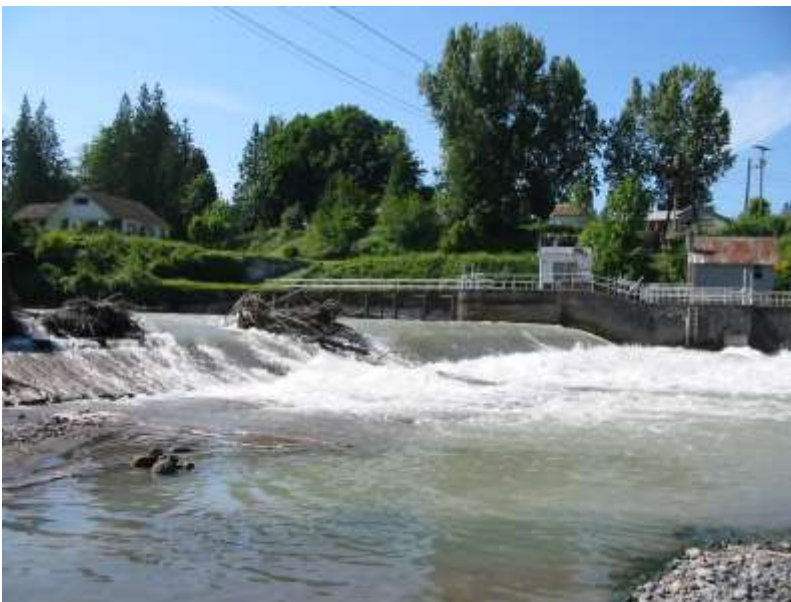
Figure 7.18 – White River Buckley Diversion Dam
