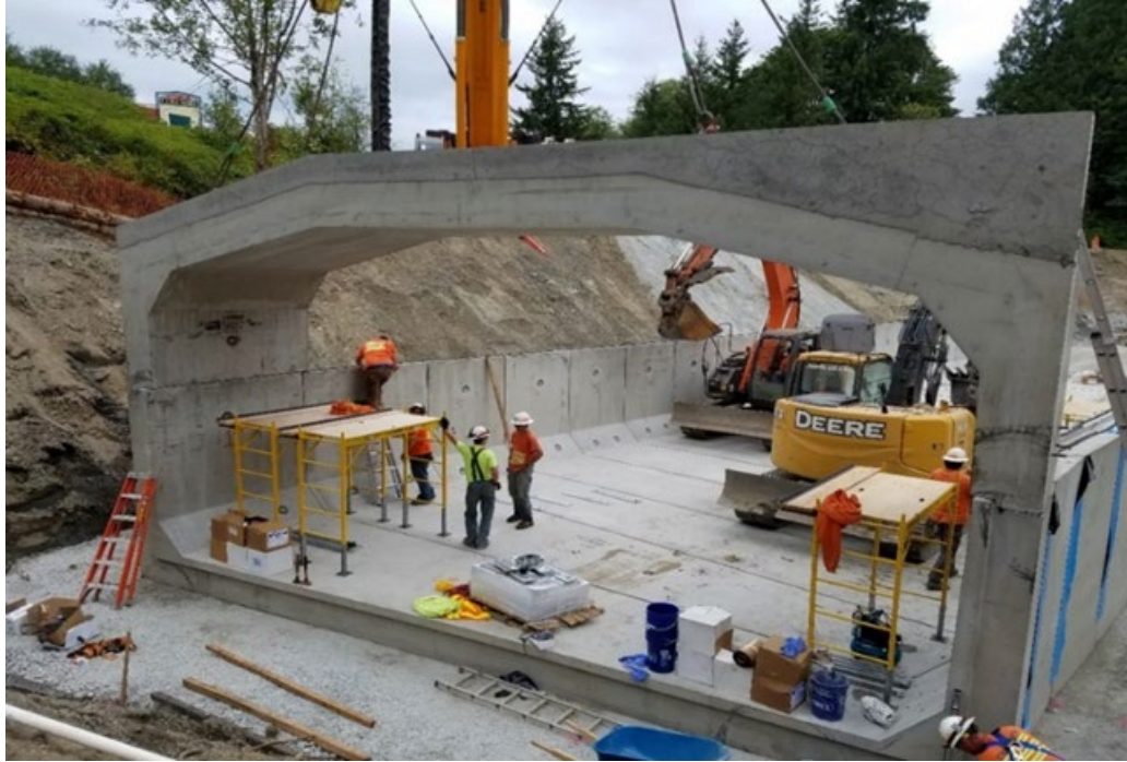
WSDOT Std. Plan E-20.10 – Buried Structure Split Box
